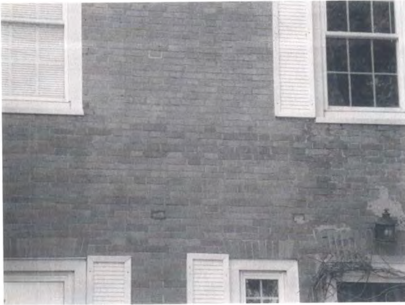
Red brick in Flemish Bond construction Brick headers over window and door openings
