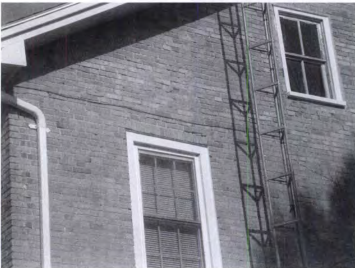
West gable end showing very simple brick header over window opening as well as simple, unadorned soffit and eaves
