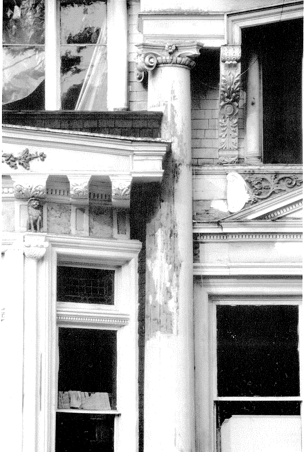
Conservation in progress, detail by detail.
