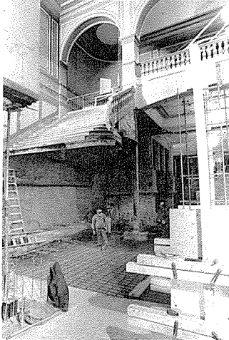
While most structures are supported from beneath, there are many instances of structures suspended from above or cantilevered from one side. Every structure must be fully understood, with the help of expert advice as required, before it can be repaired or altered.
