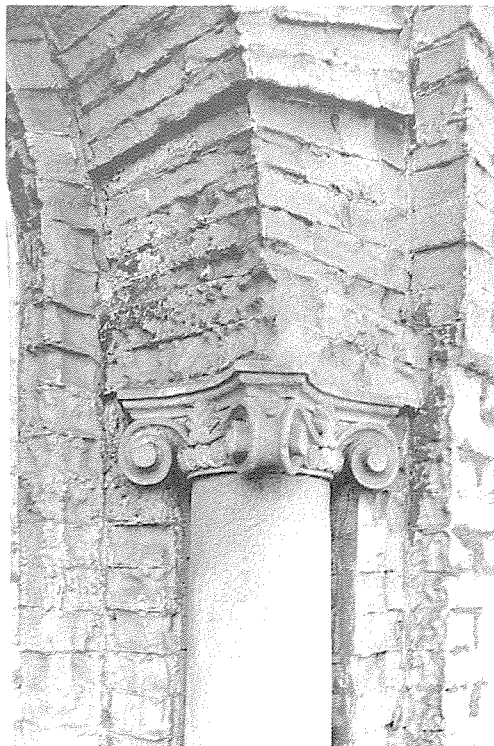
A low-pressure water-soaking for limestone — slow but effective, so long as the water can evaporate without harming the interior of the walls (above). Sandblasting on the other hand produces harrowing results — and here it did not even remove all of the paint (right).
