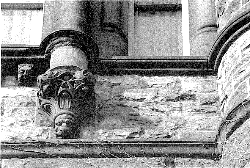
Romanesque and Classical styles of carved stone ornamentation — the rusticated styles gained particular popularity in the late 19th century for the pragmatic reason that they weathered and aged more graciously than the precise and polished styles.
