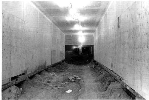
When conservation work involves major disruptions of interior spaces — in this case the excavation of a new basement — it is vital to protect finishes from damage with interior “hoarding” (above and right).
