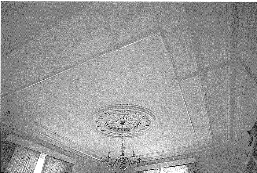
An ornamental plaster ceiling worth preserving (above): though the sprinkler system's pipes interfere with it visually, they have not actually caused much physical damage; perhaps they may be concealed in the course of future work. And a woodwork detail worth preserving (right): sliding wood doors with overlapping covers that conceal the slots when the doors are fully retracted.
