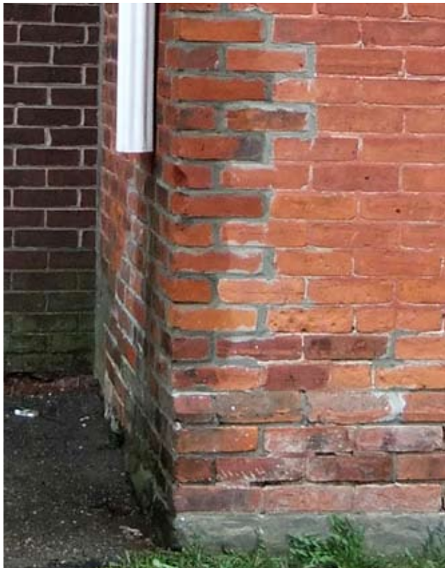
Inappropriate repointing
