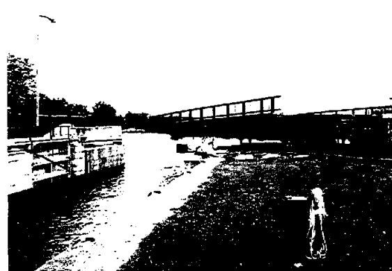
Figures 8-9: Above – Hogs Back Swing Bridge, Rideau Canal System, Ottawa, showing the asymmetrical structure swinging from one end only, and partially open (Wikimedia Commons, July 2006.). Left – Little Current Swing Bridge, Northeastern Manitoulin and the Island, Ontario (Wikipedia).
