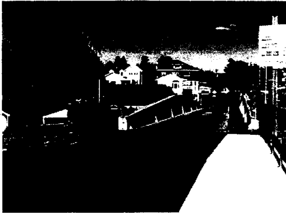
Figure 7: Above – Current bridge deck showing the steel grate deck of the vehicle lane on the left and the pedestrian walk on the right, viewed from the west (photo E. Tumak, Sept. 2013).
