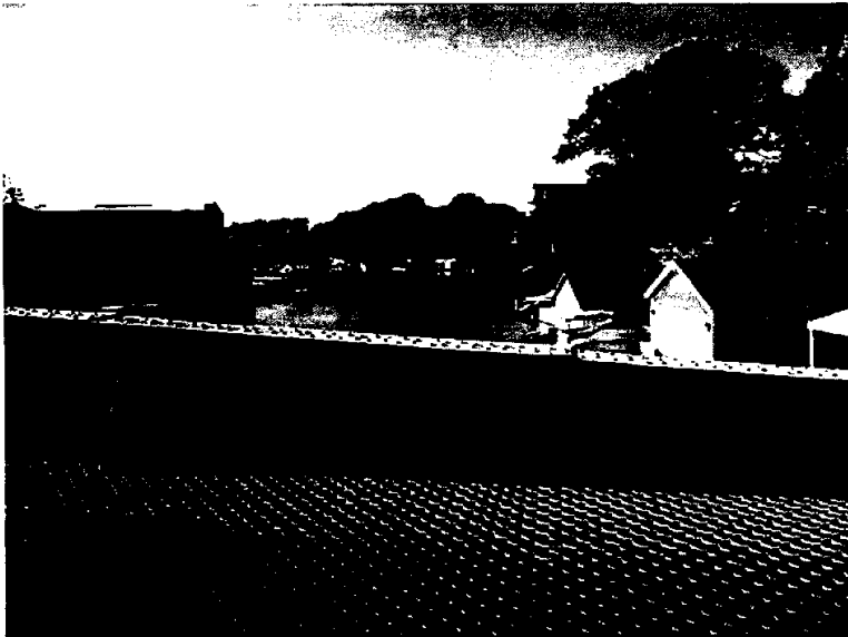
Figure 6: View from the bridge looking north up the Gananoque River showing the bridge deck steel grill of the vehicle lane and one of the stiffening plates (photo E. Tumak, Sept. 2013).
