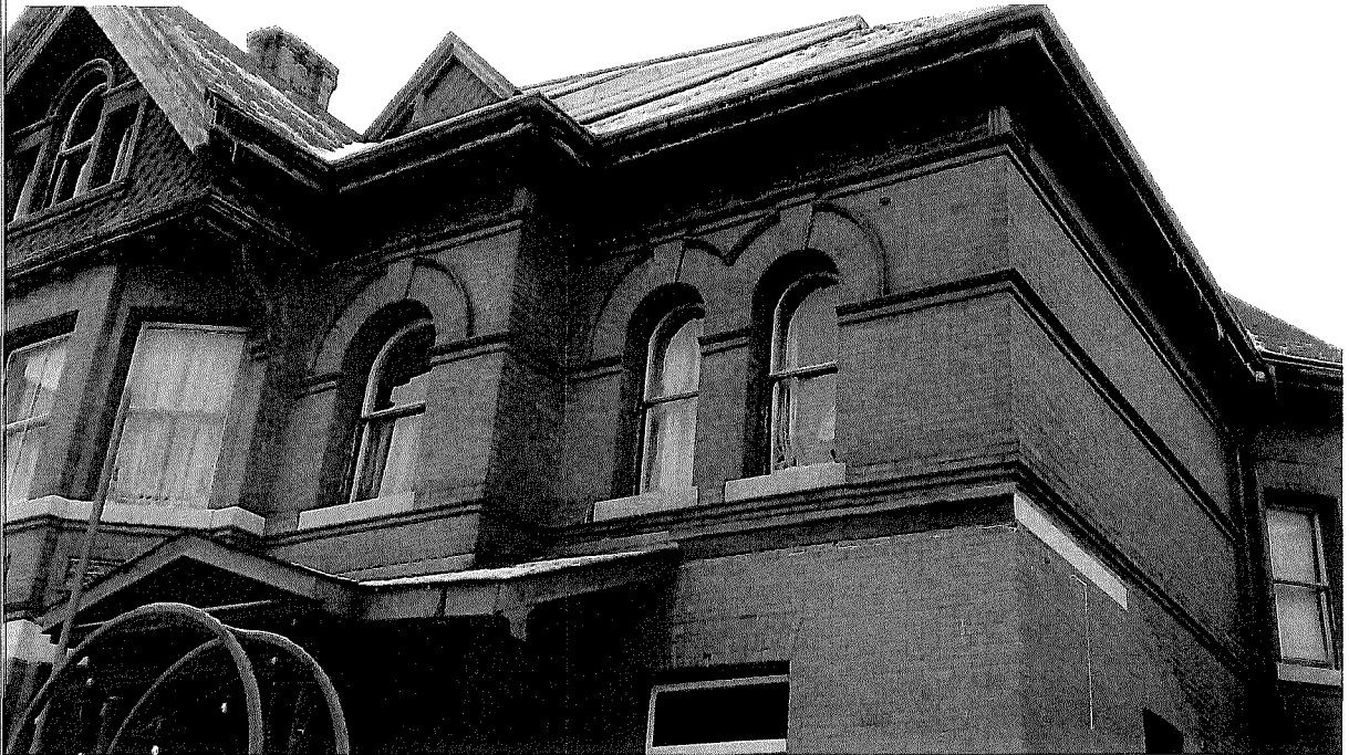
Figure 18: Detail of the second level windows at the west side of the front, highlighting the voussoirs and the terra cotta panels above (E. Tumak, Jan. 2020).
