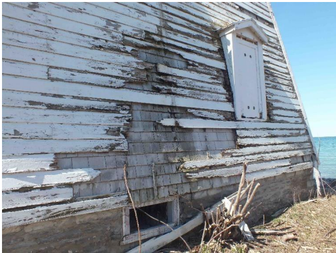
Shingle-cladding visible below later horizontal wood siding, before both layers were covered with fibre cement siding by Parks Canada (Photo: Marc Seguin,
