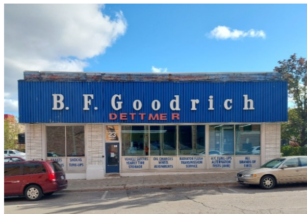
Figure 29: Dettmer Tire building with current cladding (A.S.I. 2023).
