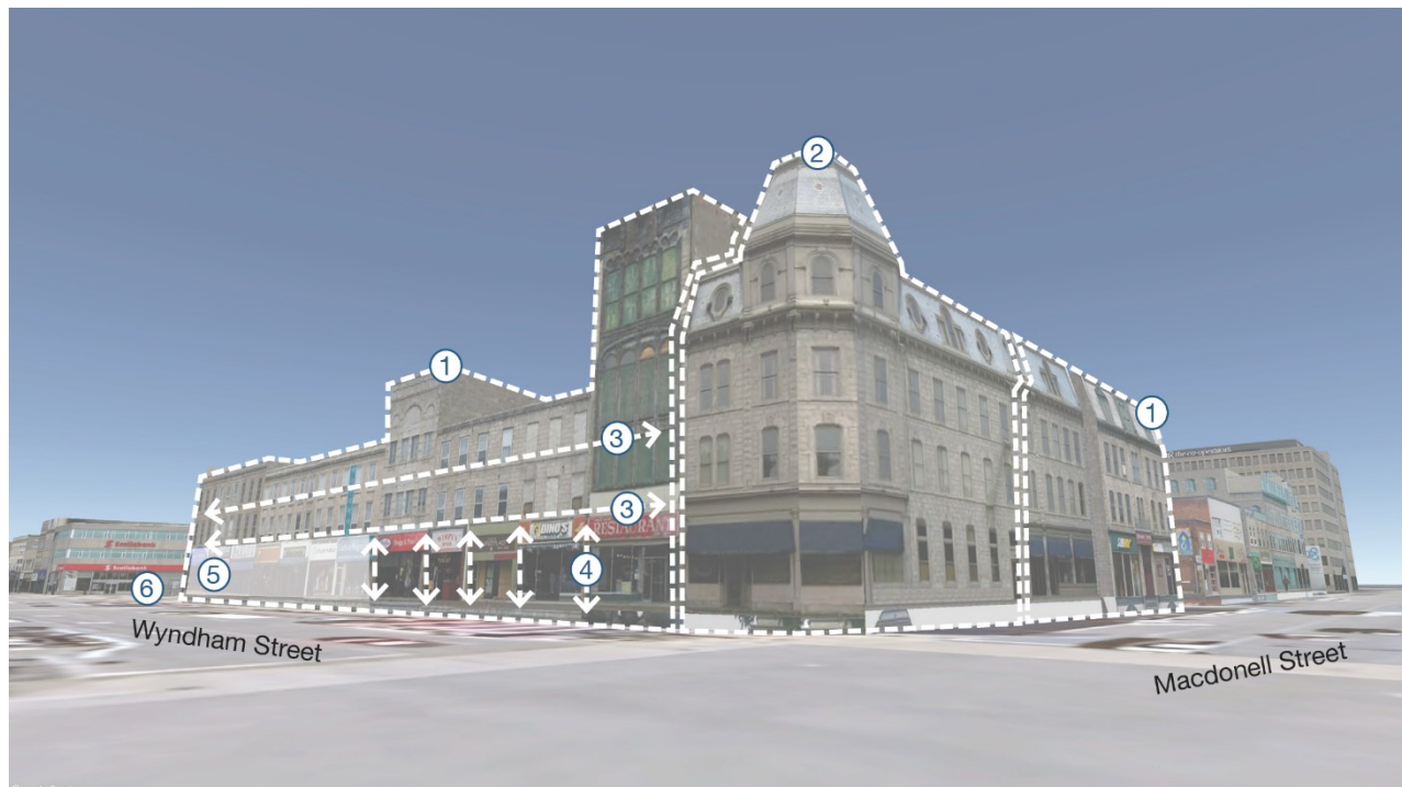
Figure 28: Example of a Contributing Property (Fotenn, 2025).
