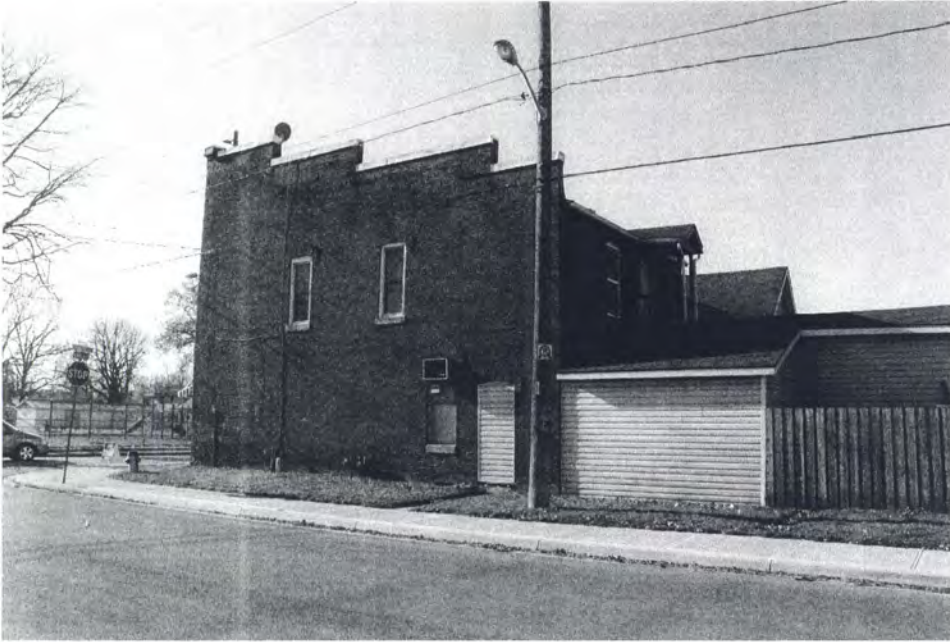
Stepped parapet side.
