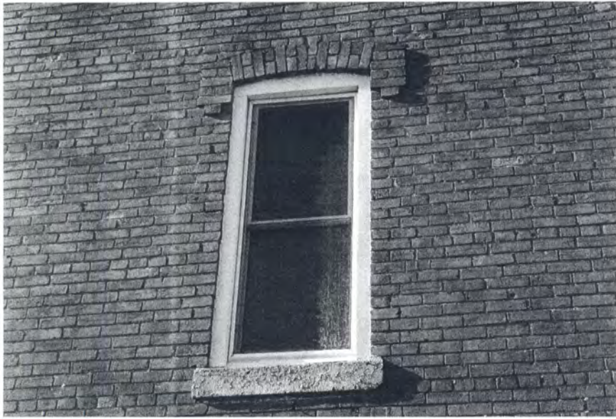
Stretcher bond construction with irregularly spaced header course, brick voussoir, lug window sill, original window placement and opening.
