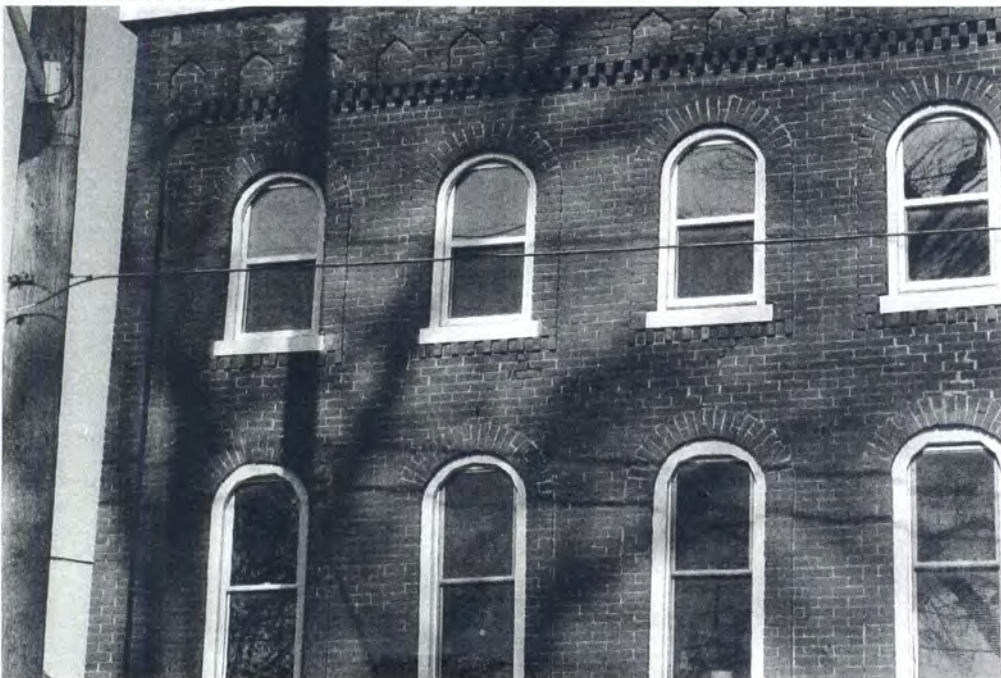
Decorative frieze, dentillated detail, arcaded windows with arched brick headers and dentil detail under sills.
