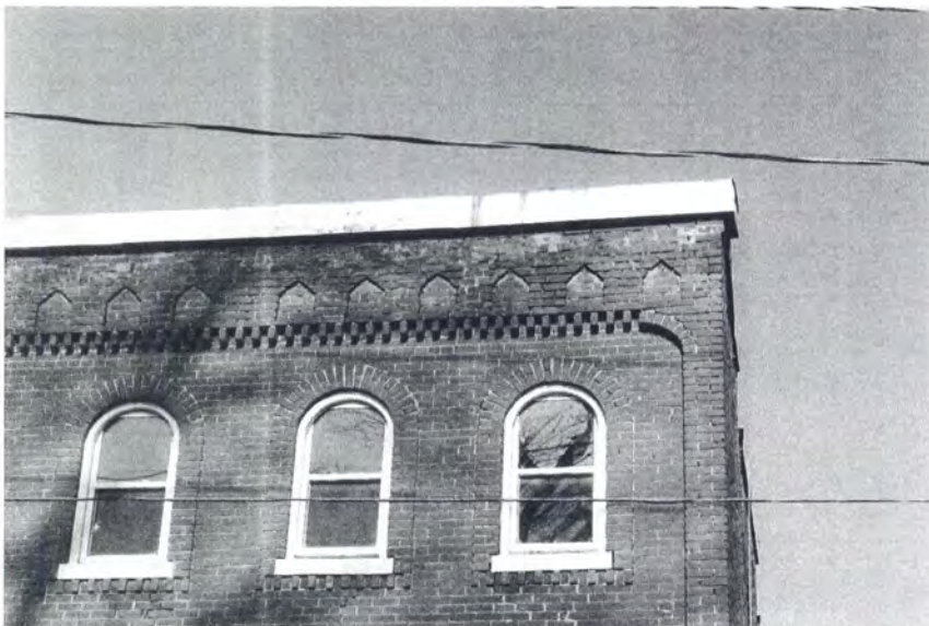
Decorative frieze, dentillated detail, arcaded windows with arched brick headers and dentil detail under sills.
