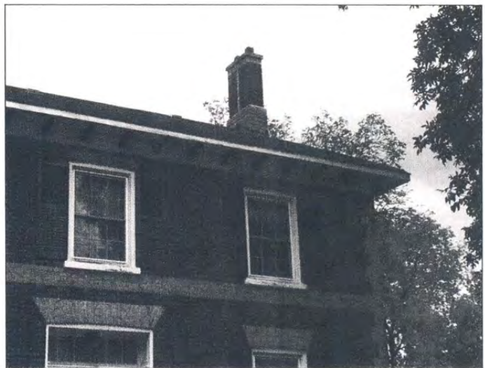
Photo #10 Buff coloured brick on lintels, quoin corners and banding running along beneath second story windows
