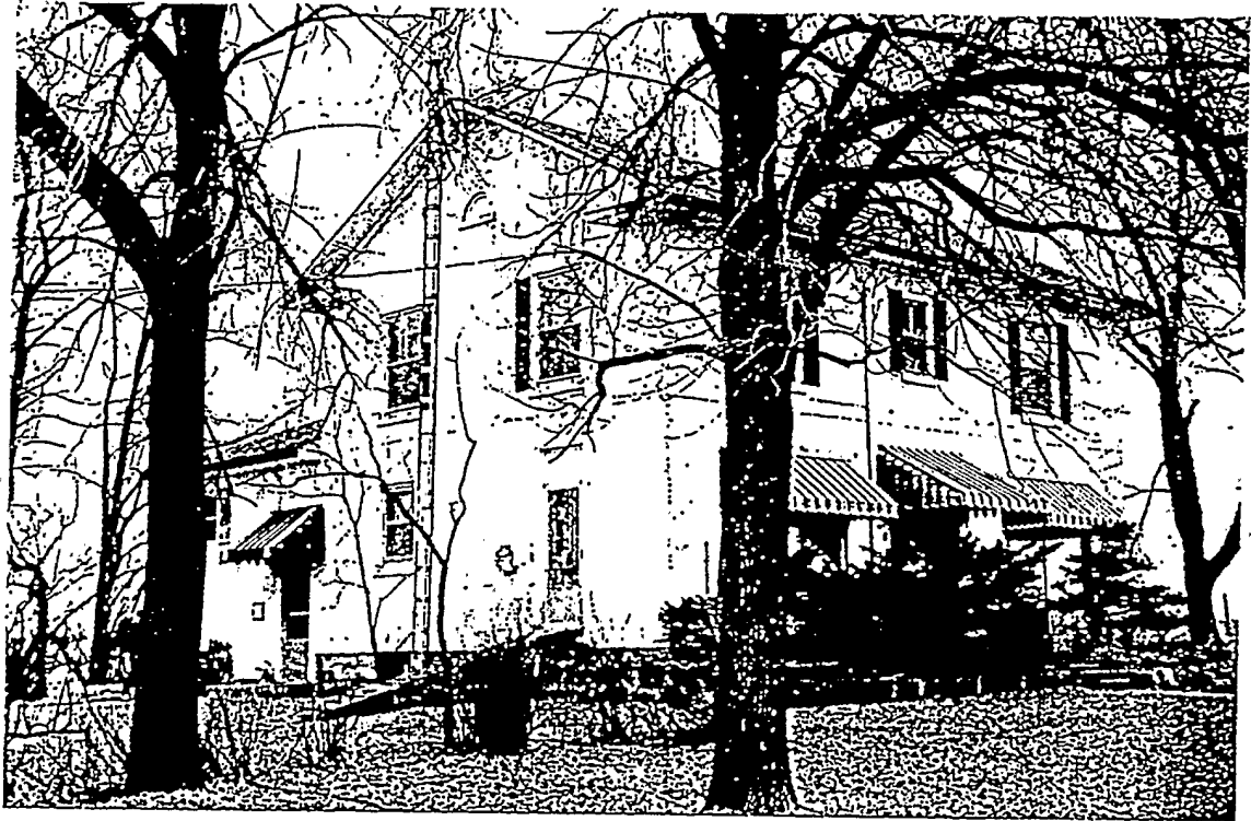
Bradburn house, showing window alterations and rear addition.
