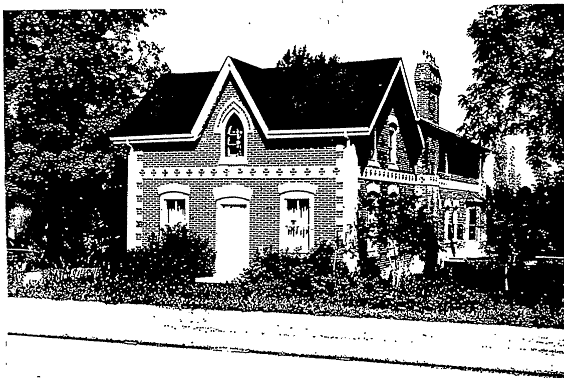
The Francis Button House 9221 Woodbine Avenue Hamlet of Bliss Corners Buttonville Heritage Study Area
