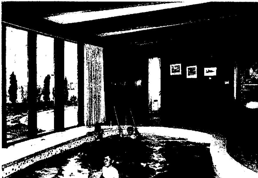
Figure 12: Indoor pool of the roundhouse; timber beams and picture windows visible ( Ontario Homes & Living 1965, pg.8).
