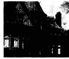
8. Hipped roof dormer with slight bellcast
