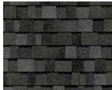
70. 3-tab asphalt shingle roofing. (Source: Roofpedia)
