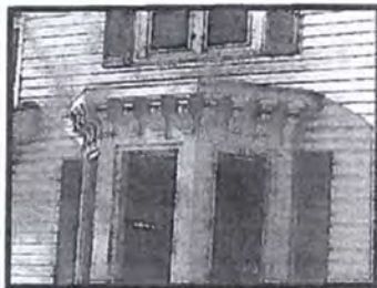
Bay window upper detail- brackets
