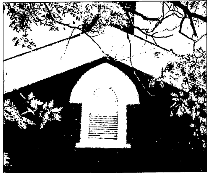
Photo 5 - Gothic vent in Gable End and Common Bond brick pattern.
