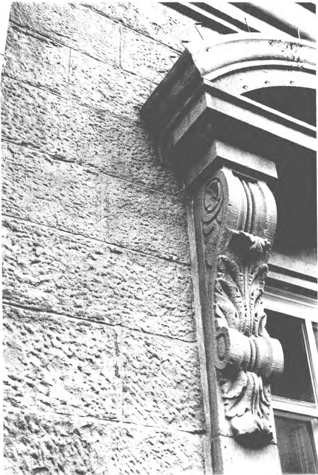
Detail view showing pediment bracket and surrounding masonry of Welland County Courthouse.
