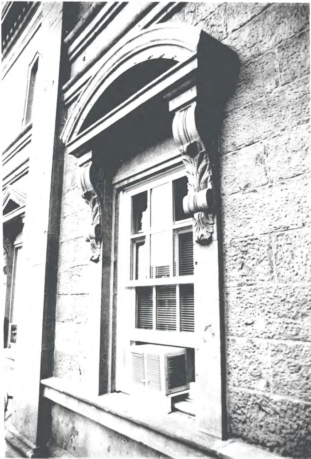
Detail view of second floor window on West facade showing pediment, bracket and frame of Welland County Courthouse.
