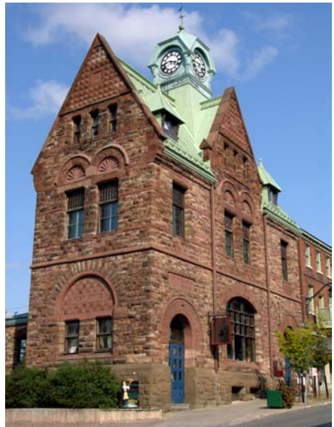
Almonte Post Office
