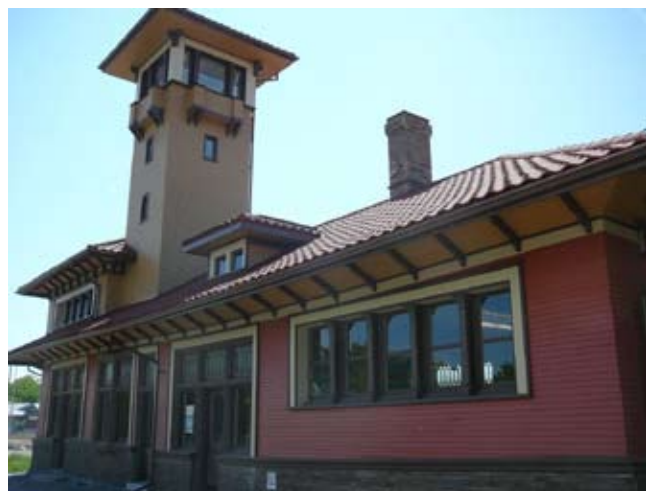
Allandale Station, Barrie before and after restoration work
