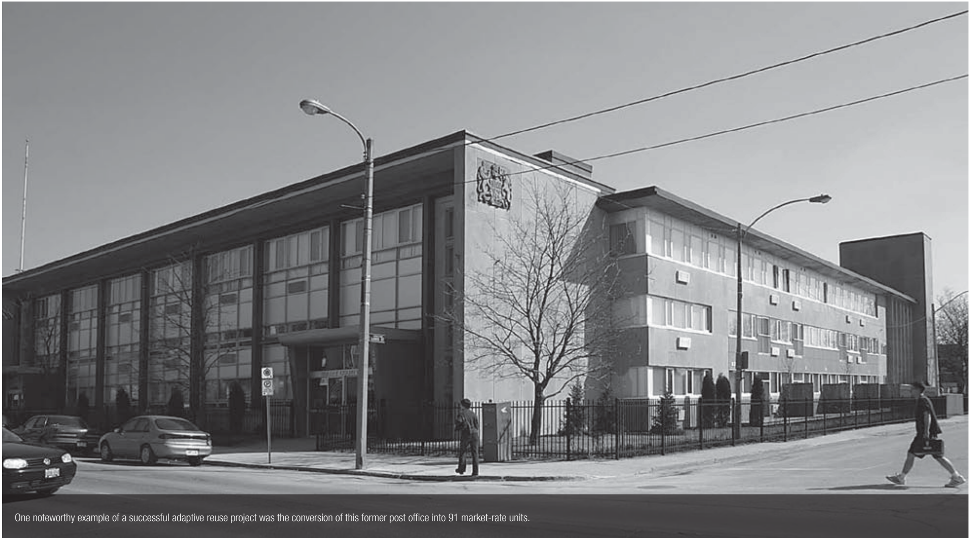
Because the post office was outfitted with heavy sorting machinery, the building's concrete floors had to be heavily reinforced. This feature ultimately enabled the basement to be converted into a parking garage, an appealing feature for this project.
