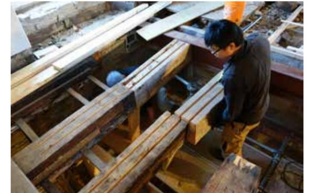
New and old timber sections prepared for insertion of reinforcing steel plates.
